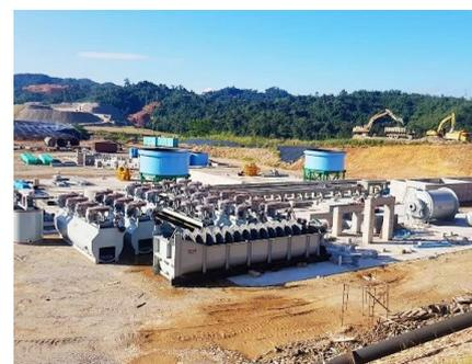
*Machineries for CNMC's proposed flotation plant, which will be able to process about 500 tonnes of ore a day to monetise silver, lead and zinc resources*
